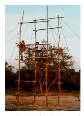
After raising and securing tower sections with guy ropes, lash on bracing poles and crossed sticks, starting from the bottom, and working your way up. Build and use an improvised ladder, if needed.
