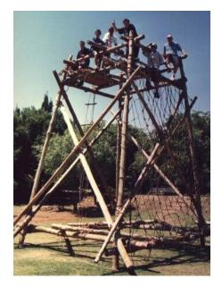
Twelve-Pole Tower: This tower is very quick to assemble, and is a very stable design (as long as the base is made wider than the top), but it requires twelve long poles to construct.
